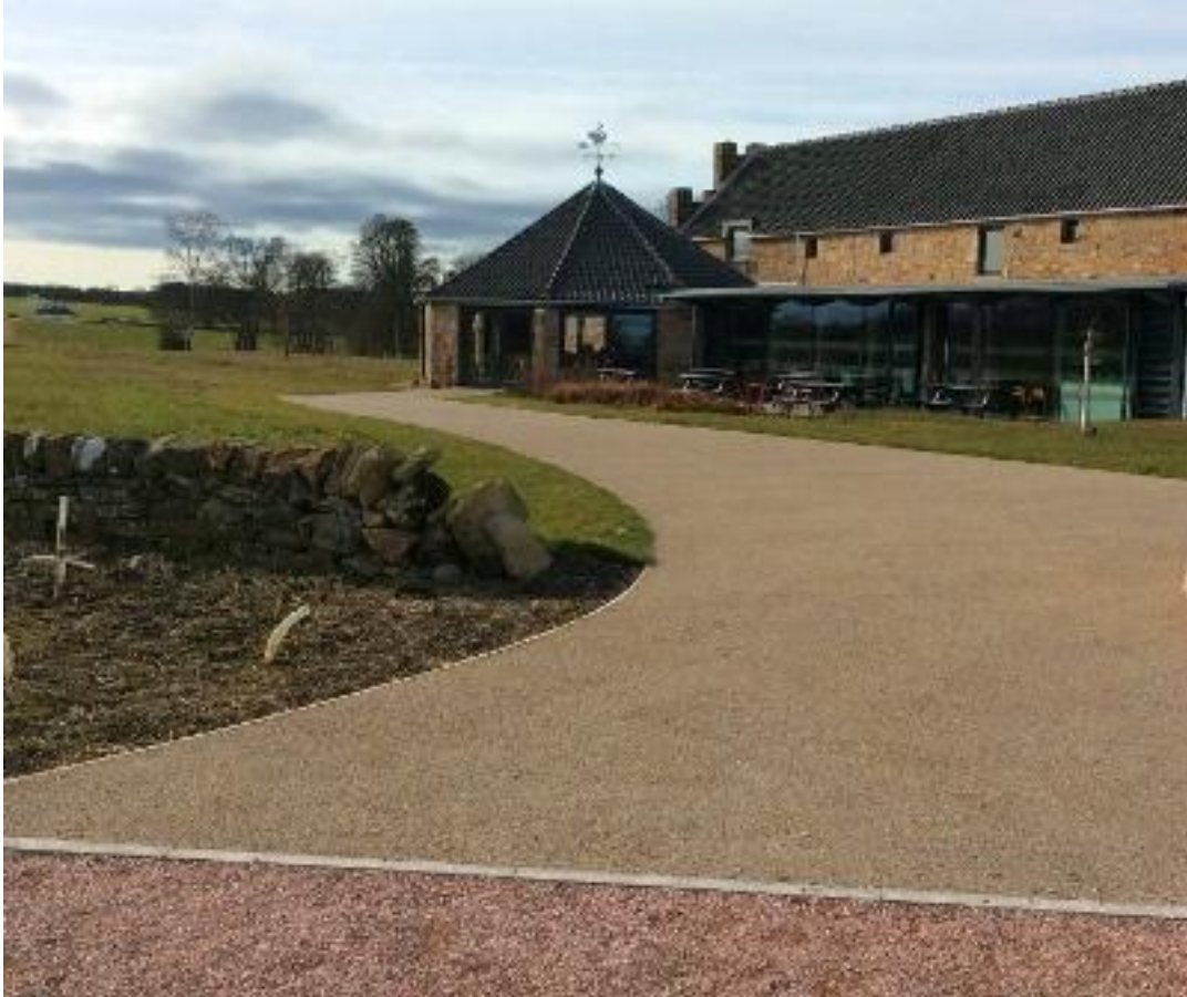
walkway to entrance, reception and outdoor space
