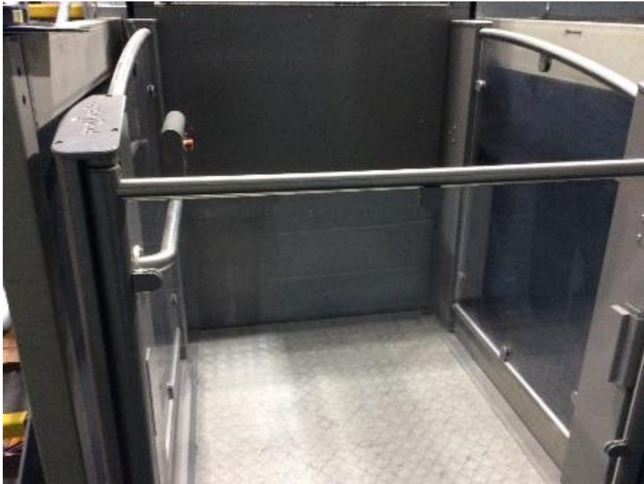
photo above: platform lift
