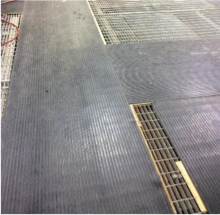
photo above: walkway on upper level (rubber matting)
